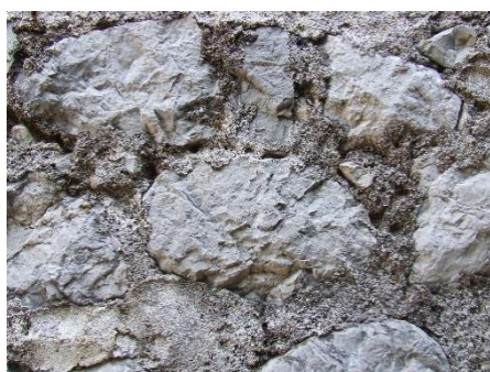
Figure 20. Front façade walls were built using the highly regarded fine stone from Strp and Lipci quarries.
