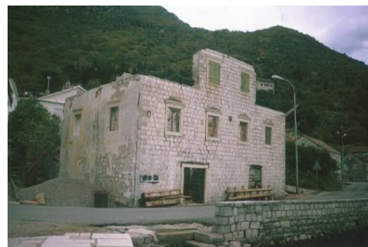
Figure 31. The façade had to be taken down due to the forced protrusion.
