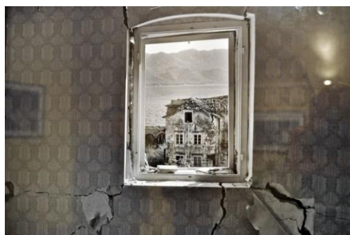
Figure 2. Openings in the walls (doors, windows) showed their vulnerability in the 1979 earthquake.
