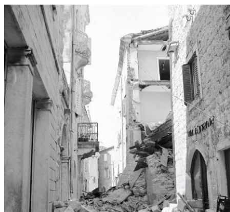
Figure 1. Collapse of row houses in urban environment (Kotor).
