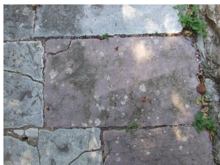
Figure 19. Less regular shaped blocks on the lateral façade from Strp and Lipci quarries.
