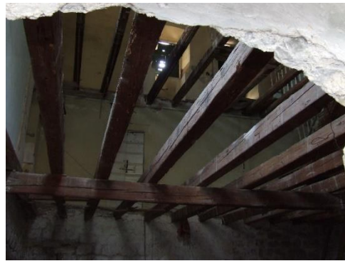
Figure 15. Transversal beams had the function of tie-rods.
