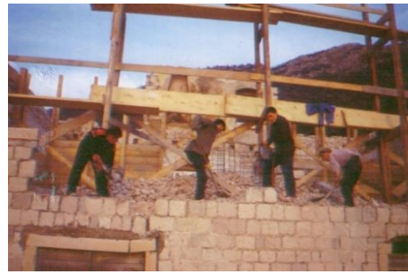
Figure 32. The façade had to be taken down due to the forced protrusion.
