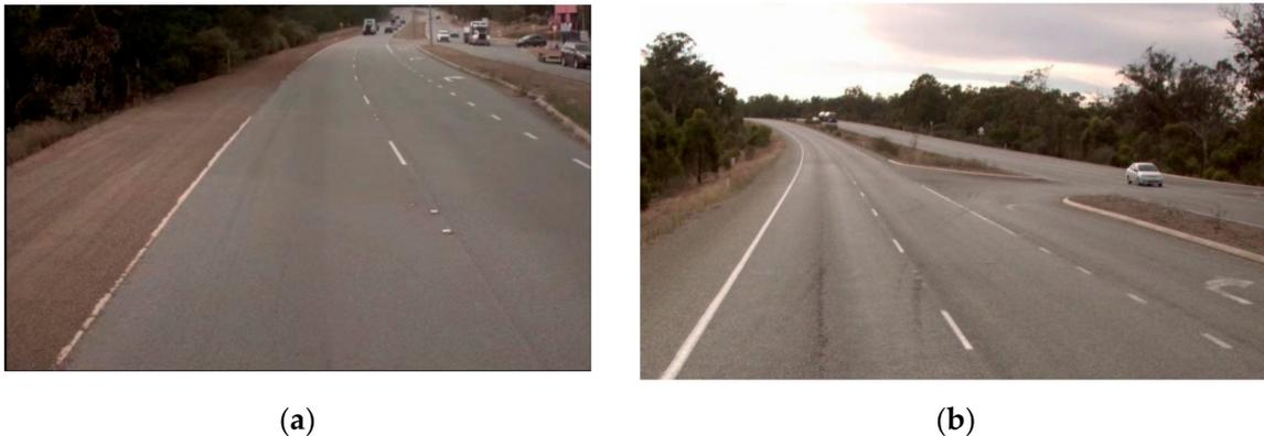
**Figure 1.** Examples of pavement markings in poor condition. (a) Edge line (left side) is worn down and even missing; (b) turning arrows and continuity line (right side) are blurred.
