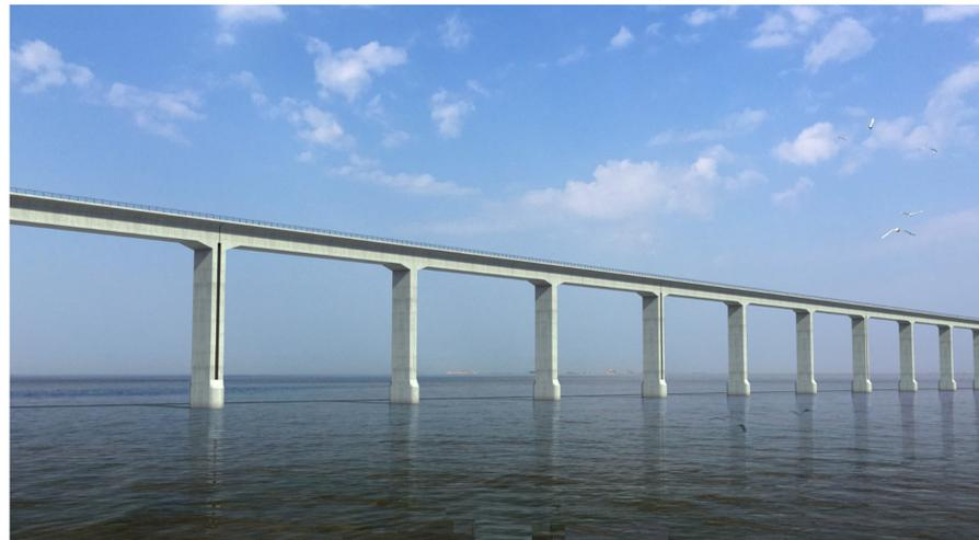
Figure 4. Design rendering of the integral rigid-frame bridge of the Fuzhou–Xiamen high-speed railway (HSR).
