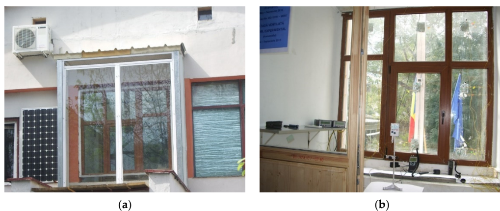
Figure 1. View of the double-skin façade: (a) from the outside of the building and (b) from the inside of the interior room.
