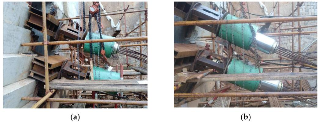
Figure 16. The schematic diagram of active control. (a) Jack tension initial state; (b) Jack tension state.
