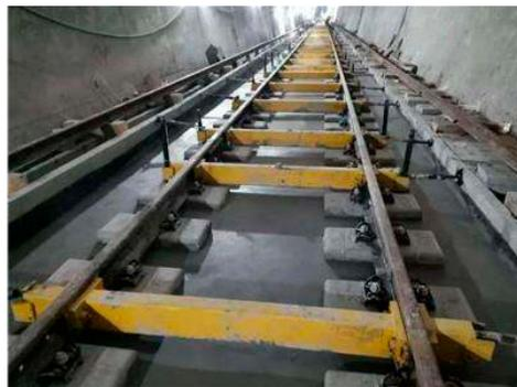
Figure 6. LVT construction site in the tunnel.
