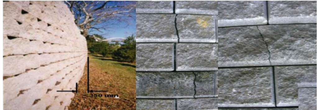
Figure 1. Excessive deformation of the retaining wall [6].
