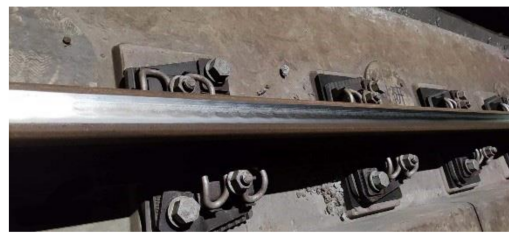
(a) Short pitch corrugation on the inner rail
