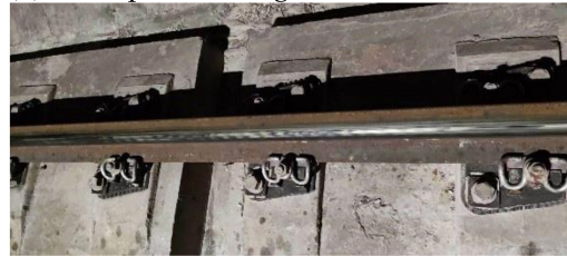
(c) Side corrugation on the outer rail
