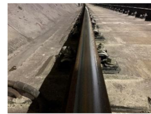
(b) Long wavelength corrugation on the inner rail
