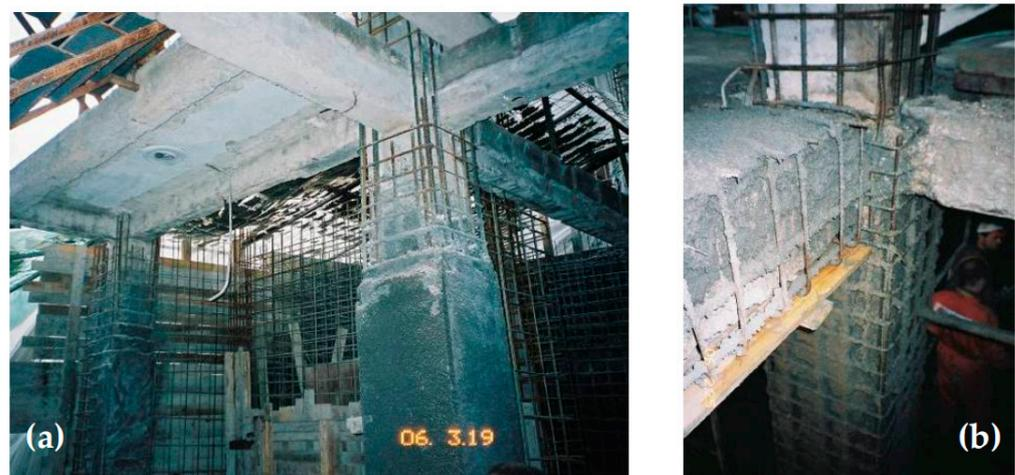
**Figure 1.** (a) RC jacket of columns employing shotcrete (gunite). (b) RC jacket of column and beam at the region of their joints employing shotcrete (gunite) [13].
