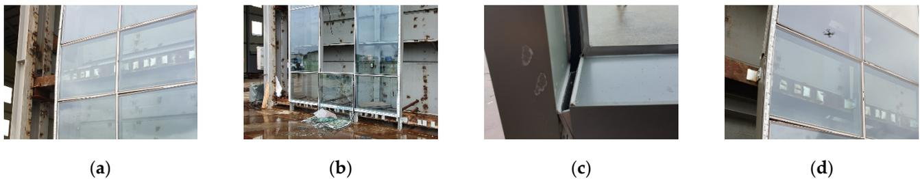
**Figure 4.** Main vulnerabilities of non-seismic curtain wall: (a) external weather sealant breakage; (b) glass fallout; (c) curtain wall frame breakage; (d) expansion joint breakage.
