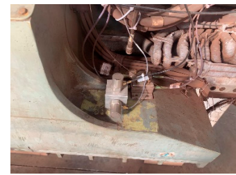
(c) Vertical displacement and vibration test of bridge
