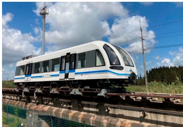
Figure 5. Coupled low-to-medium-speed maglev train and steel beam system in the field test.
