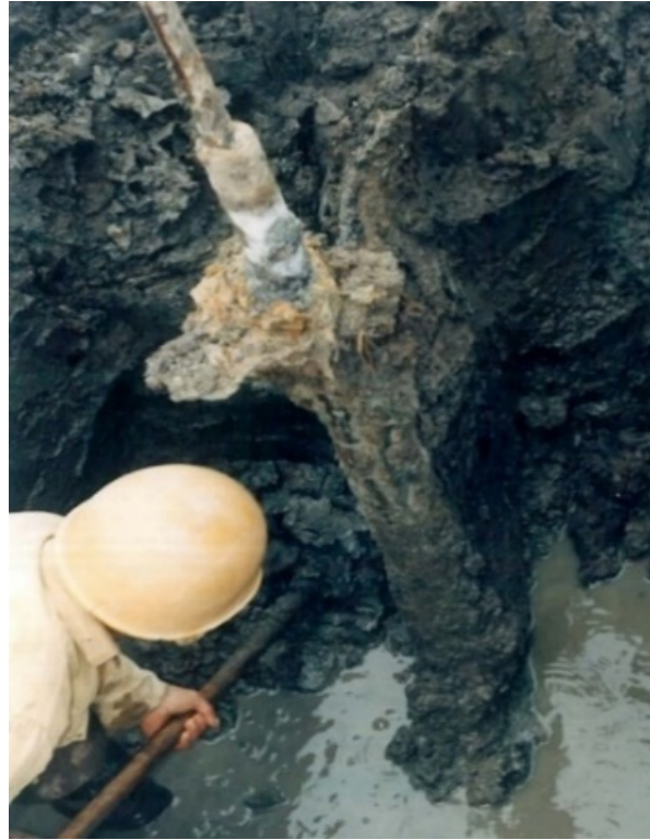
Figure 2. Single bar reinforced micropile after the first phase of pressure grouting using a sleeve pipe.
