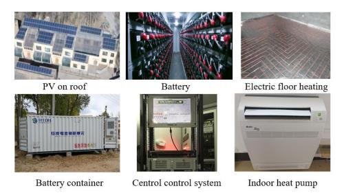
Figure 25. Photos of key equipment of the microgrid.
