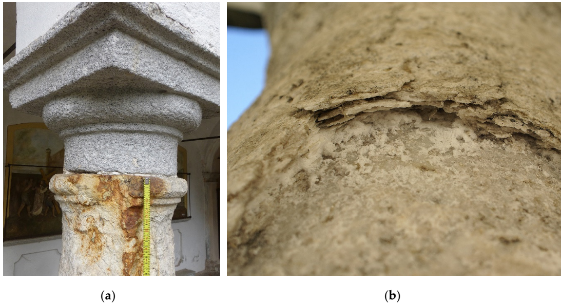
Figure 3. Examples of erosion (a), exfoliation and detachment (b) problems in stone columns of the Via Crucis portico. The reference lexicon is that of the "Ente Nazionale Italiano di Unificazione" (UNI) Standard rules 11182:2006.
