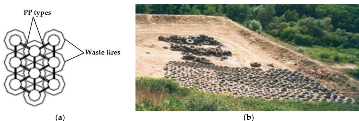
Figure 3. (a) Scheme of tire junction with PP- polypropylene tape, and (b) tire mattresses built in the landfill slope.
