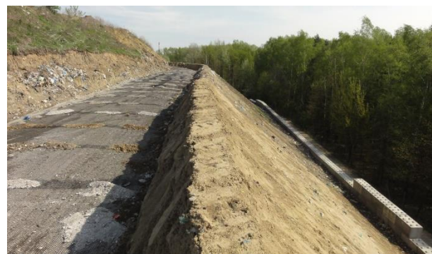
Figure 2. (a) Geometry of uniaxial geogrid and (b) landfill slope reinforced with geogrid.
