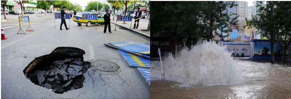
**Figure 1.** Pavement collapse and pipe burst caused by cracks in concrete pipes.
