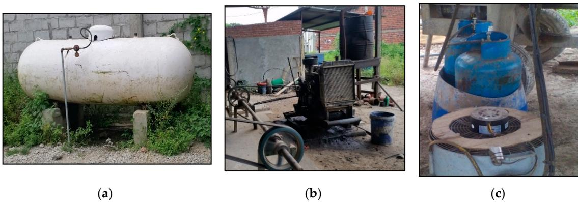
**Figure 9.** Types of fuels used as a heat source: (a) liquefied petroleum gas (LPG) tank for industrial use; (b) Diesel used for the operation of the generator; (c) LPG cylinder for domestic use.
