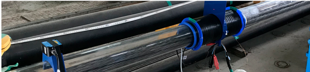
Figure 7. View of external PSC tendon installed for measurement test of sectional loss by the Total Flux Leakage (TFL) method.
