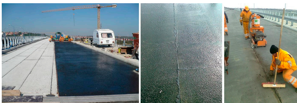
Figure 3. Longitudinal joints in a mastic asphalt pavement constructed in stages [33].
