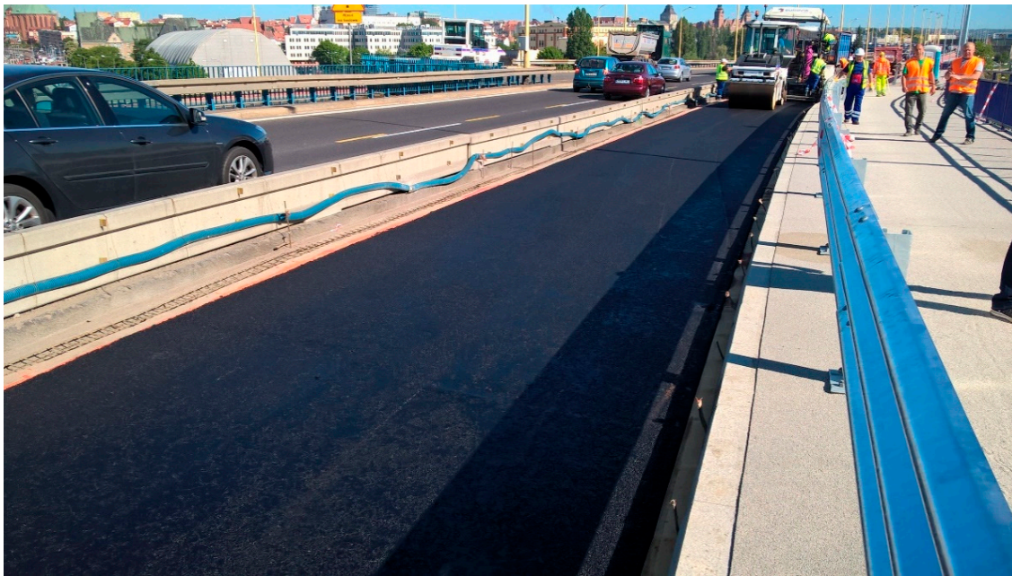
Figure 15. Compaction of the SMA-MA 8 PMB 45/80-65 protective layer.
