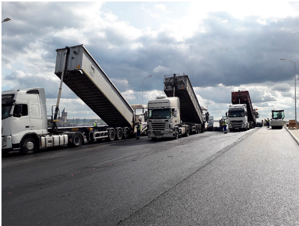
Figure 18. Placement of wearing course of SMA 11 PMB 45/80-65 mixture.
