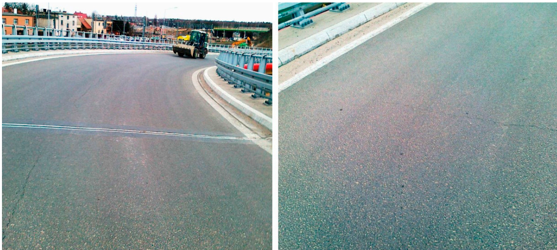
Figure 4. Distressed wearing course due to shrinkage and cracking of the protective layer of mastic asphalt.
