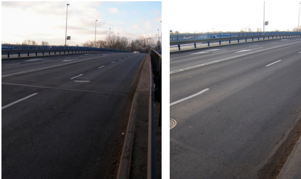
Figure 9. Condition of pavement with the protective layer made of SMA 11 mixture with increased amount of bitumen mastic on the overpass supporting Mickiewicza St. in Szczecin in year 2017 (year of completion: 2001).
