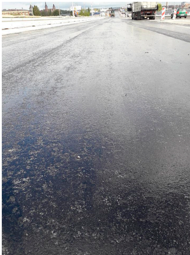
Figure 16. Surface of the SMA-MA layer after compaction.
