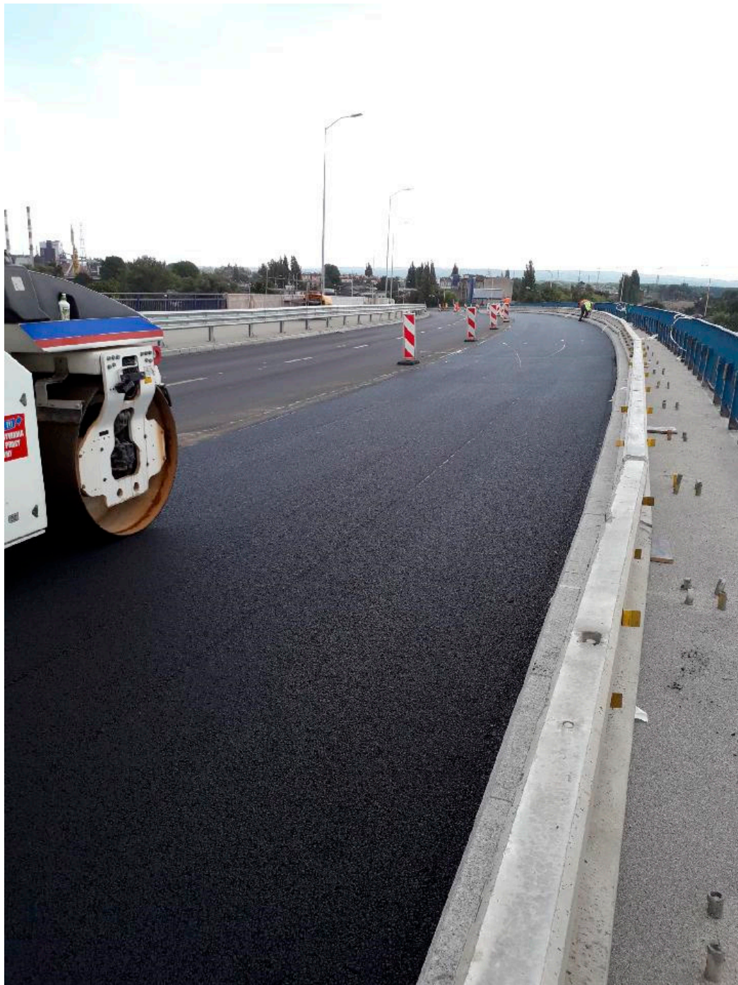
Figure 17. Compaction of binder course of asphalt concrete (AC) 11 S PMB 45/80-65 mixture.
