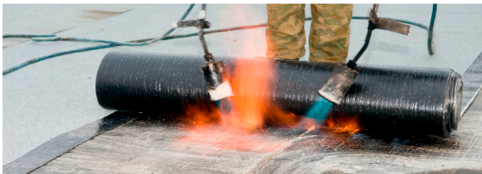
Figure 2. Application of a torch-on membrane—heating up the material with gas torches.
