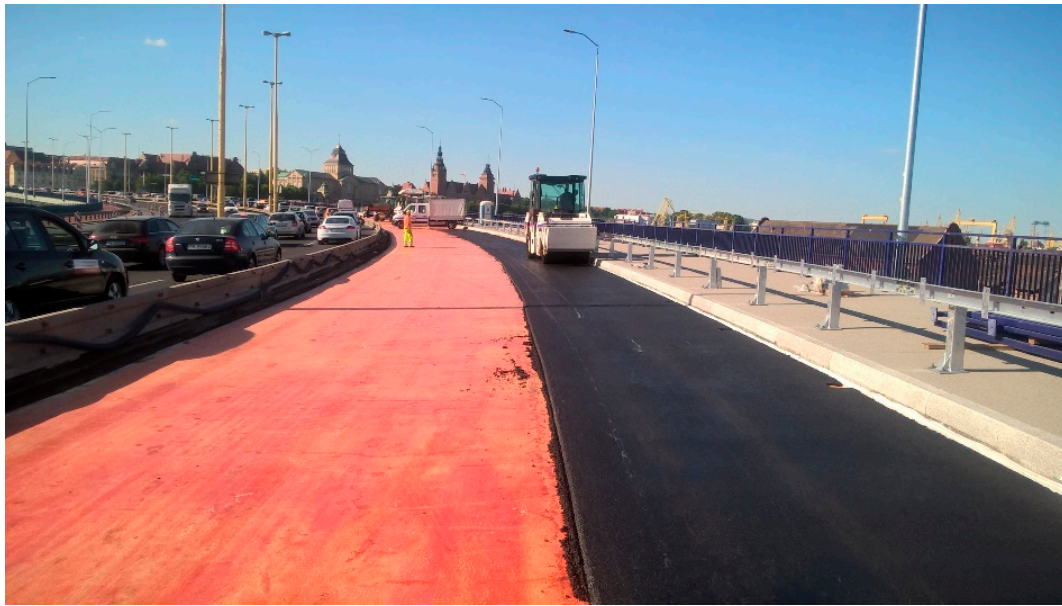
Figure 13. Methyl methacrylate waterproofing layer on the Trasa Zamkowa bridge and SMA-MA 8 layer.
