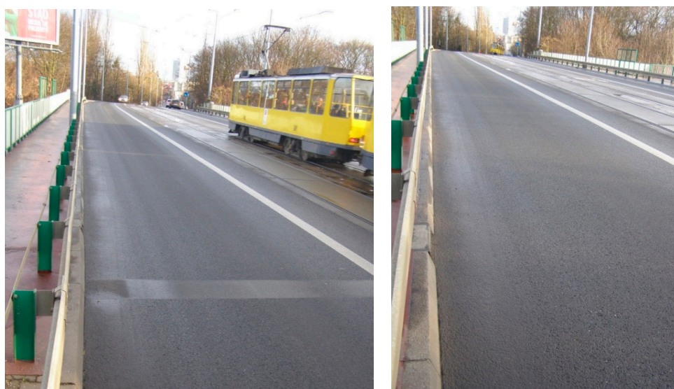
Figure 8. Current condition of pavement with the protective layer made of stone mastic asphalt (SMA) 5 mixture with increased content of bitumen mastic on the overpass supporting Mickiewicza St. in Szczecin (year of completion: 2001).
