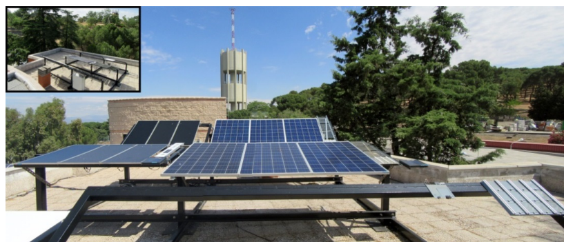
Figure 4. Panoramic view of the rooftop PV system installed for soiling monitoring.
