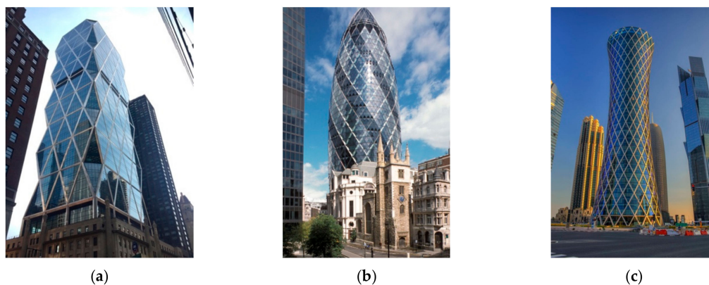
Figure 2. Examples of diagrid systems in tall buildings: (a) Hearst Tower (New York, USA), picture taken by D. Scaramozzino; (b) Swiss Re Tower (London, UK), from https://larryspeck.com/ ; (c) Tornado Tower (Doha, Qatar), from http://www.asergeev.com/ .
