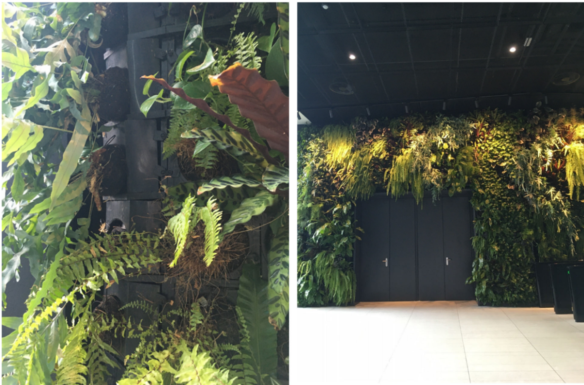
Figure 3. Modular system living wall with planter boxes in an office building (Porto Office Park, Porto-Portugal). Credits: Cristina Calheiros.
