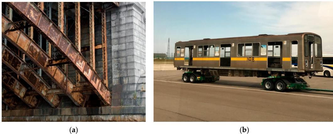
**Figure 8.** Corrosion of steel. (a) Extreme corrosion in a bridge. (b) Railway rolling stock being renovated.
