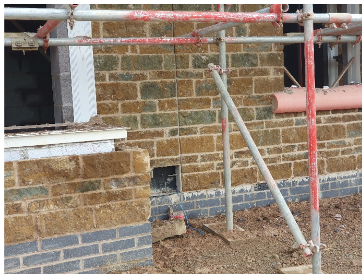
Figure 8. Example of the traditional aesthetic produced by using irregular size ironstone bricks, contrasted with the consistent facing bond achieved with the standard bricks used below, highlighting the potential for ironstone to increase material waste.
