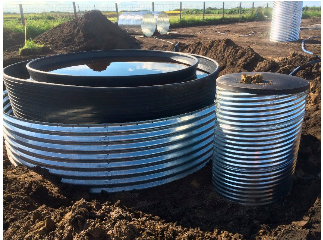
Figure 1. Mesocosm protected by steel tunnel liner and overflow tank housed within a culvert, visible during construction in 2016.
