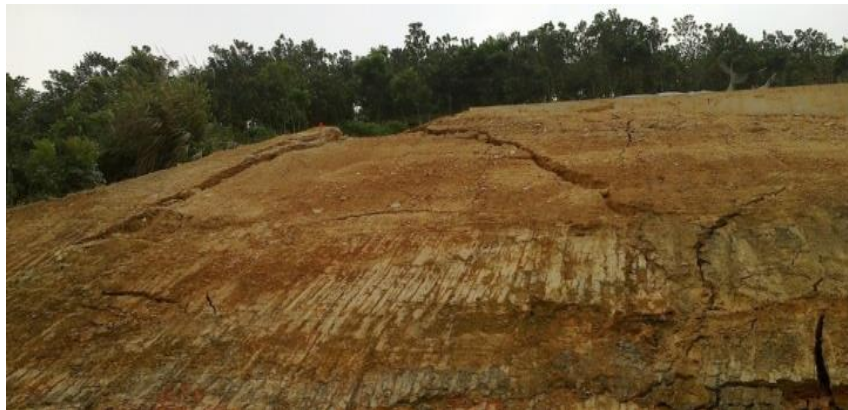
Figure 12. Landslide failure of a slope on expressway B, Guangdong, China.
