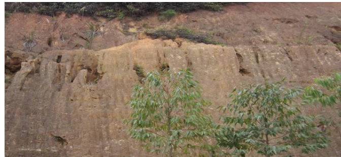
Figure 9. Weathering and surface erosion in a red-bed rock slope in South China.
