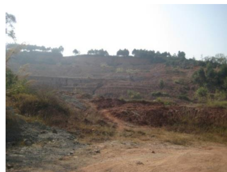
(b) Slope scouring erosion
