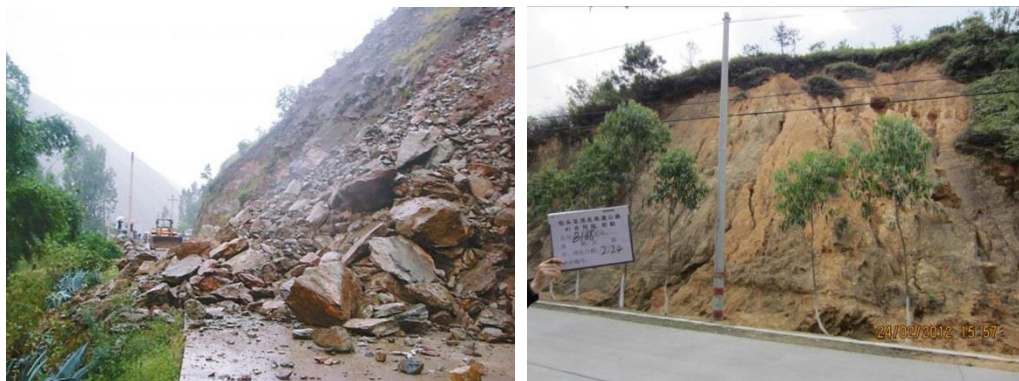
Figure 11. Collapse and falling in a red-bed rock slope in South China.
