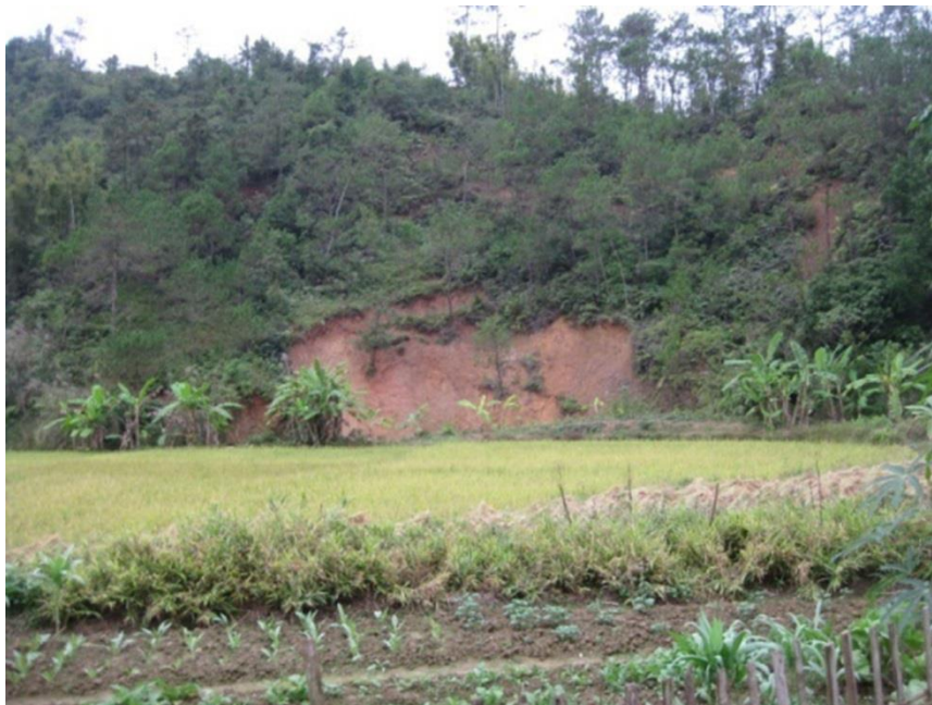
Figure 13. Landslide failure of a slope on expressway C, Guangdong, China.
