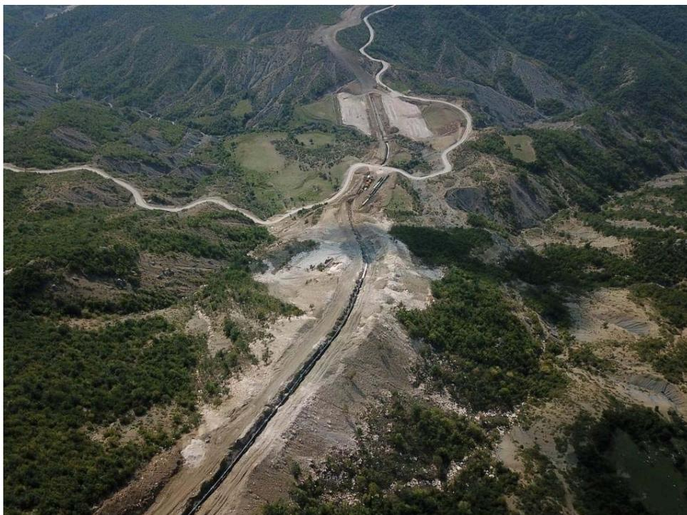
**Figure 3.** Right of Way (RoW) for major gas pipelines is a strip of land, usually between 18 and 36 m wide, containing one or more pipelines, used as access for inspection, maintenance, testing or emergency.
