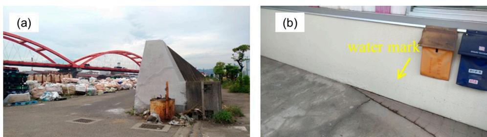
**Figure 6.** Photographs taken by the authors at Mikageishi town. (a) Coastal levee and gate at the entrance of the port storage zone; (b) Survey Point M1 (watermark is indicated by a yellow arrow).
