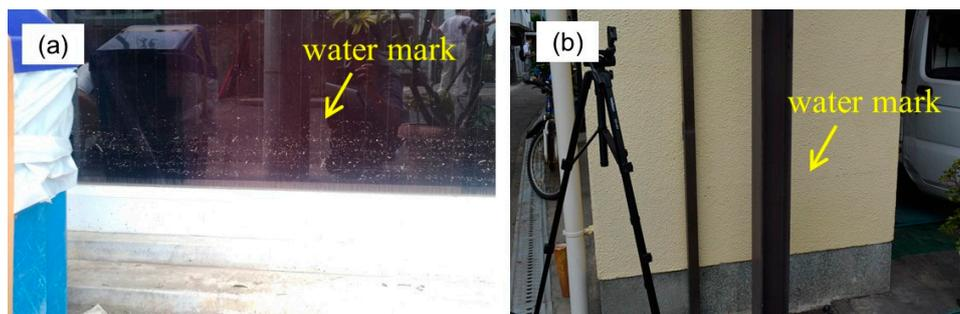
**Figure 5.** Photographs taken by the authors at Higashi-Kawasaki town. (a) Survey Point H2 (watermark on a window); (b) Survey Point H3 (watermark is indicated by a yellow arrow).
