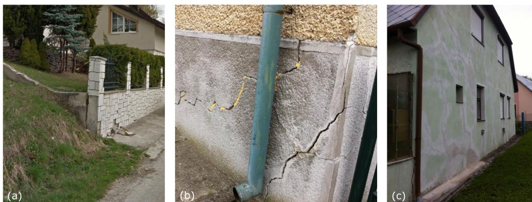
**Figure 3.** Photo-examples of structural damage in Hradec and Velka Lehotka (case study 1) caused by local slope deformations, (a) April 2012, Photo courtesy: Google Street View; (b) and (c) July 2017.
