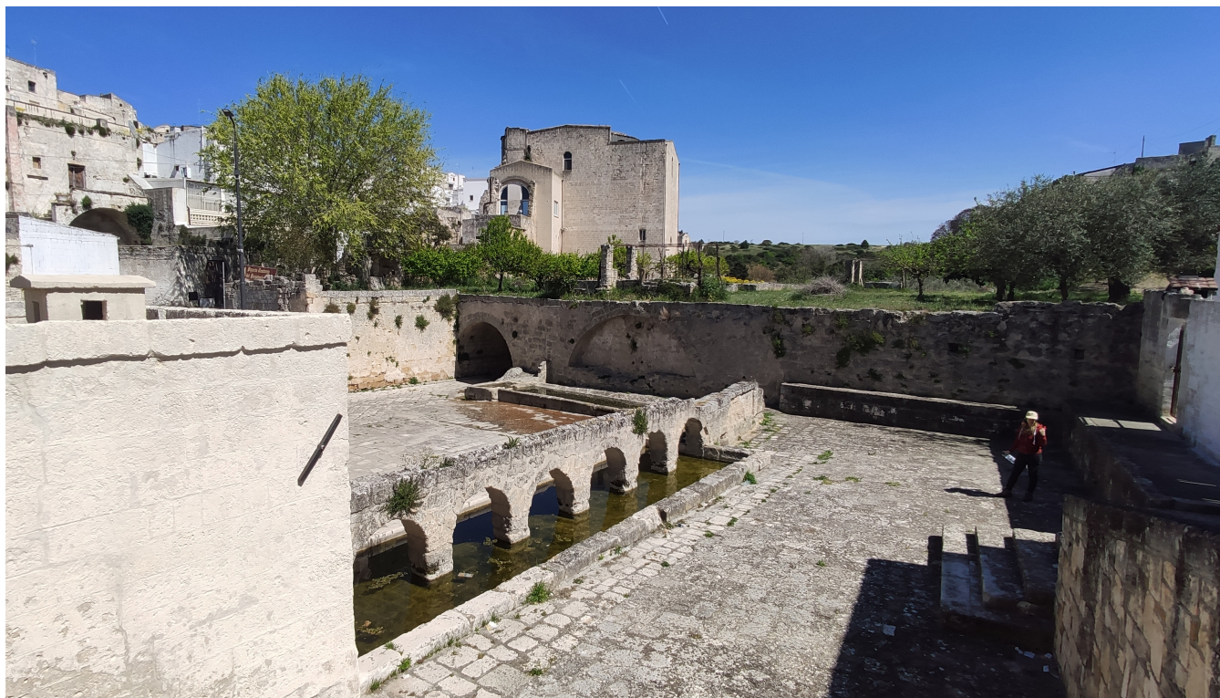
Figure 10. The second pool (at the base of the arcs) and the third one (perpendicularly located at the left end of the arcs) of the Mascheroni Fountain, built with blocks coming from the same carbonate soft-rocks dug to create rupestrian houses. The photo was taken from behind the facade reproduced in Figure 3.
