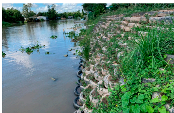
Figure 7. Condition of the riverbank two months after embankment construction using waste tyres. The image shows structural stability and successful vegetation establishment, indicating early effectiveness of the hybrid revetment system in erosion control.
