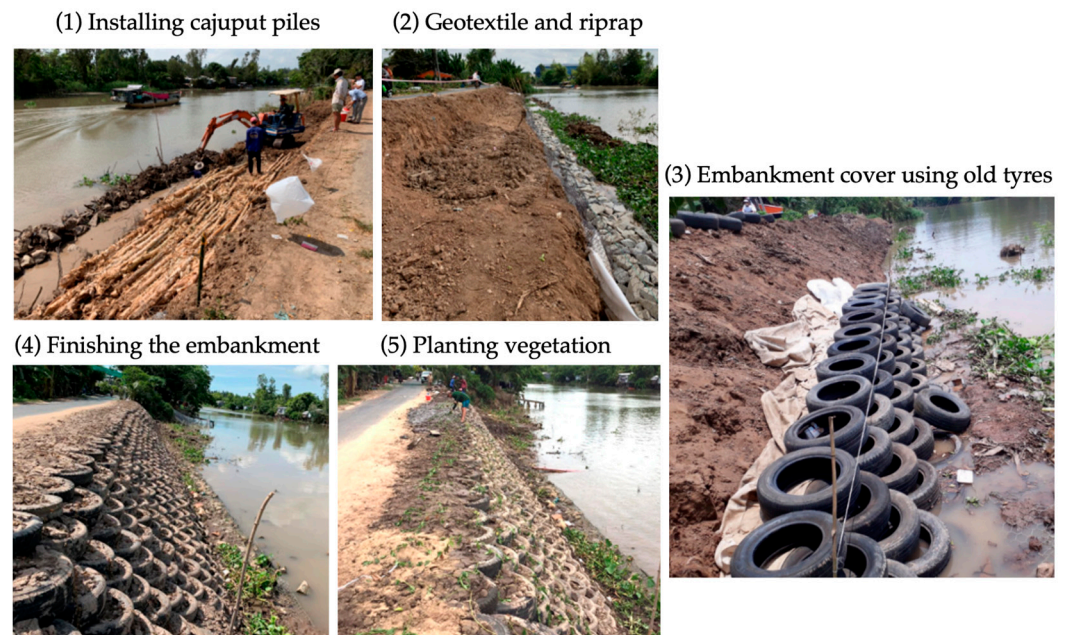
Figure 5. Step-by-step construction process of the embankment utilizing waste (old) tyres. The process includes foundation reinforcement with Melaleuca piles, placement of geotextile and riprap, installation of interlocked tyre units, earth filling, and final vegetative planting for ecological stabilization.
