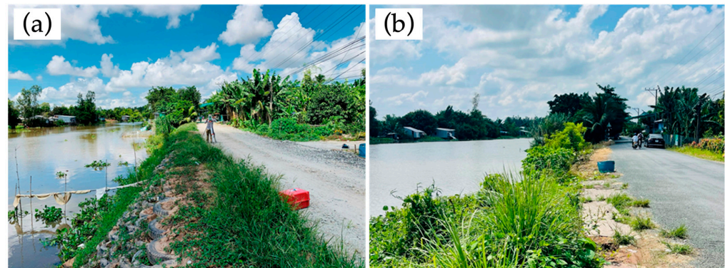
Figure 11. (a) Condition of the tyre-reinforced embankment one year after construction, showing maintained structural integrity and vegetation growth. (b) Status after five years of operation, demonstrating long-term durability despite increased road use and environmental exposure.
