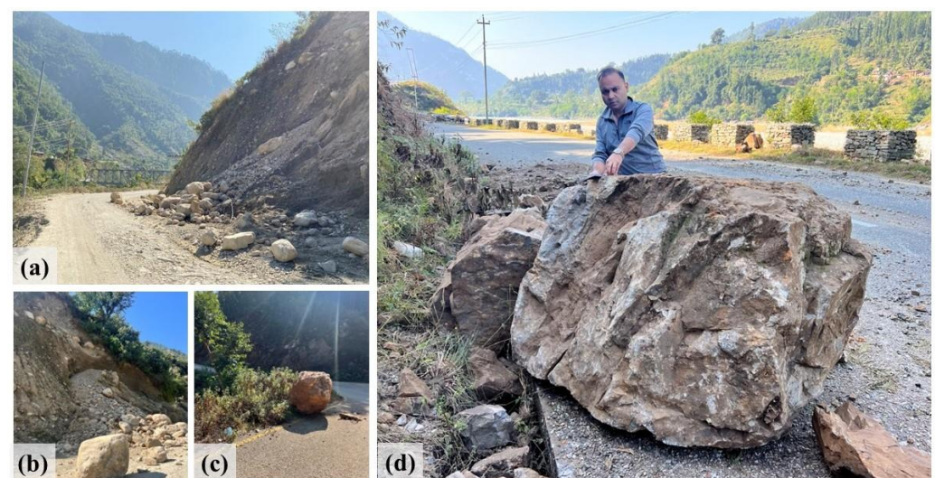
Figure 20. (a) Road obstruction due to continuous rock fall ( 28^{\circ}46'51'' N, 82^{\circ}17'33'' E) (b) medium to large size rockfall ( 28^{\circ}46'50'' N, 82^{\circ}17'33'' E) along Bheri Corridor (c) rockfall ( 28^{\circ}42'22'' N, 82^{\circ}15'17'' E) (d) large size rocks fall up to 1.73\text{ m}^3 ( 28^{\circ}42'17'' N, 82^{\circ}14'08'' E) along Midhill Highway.
