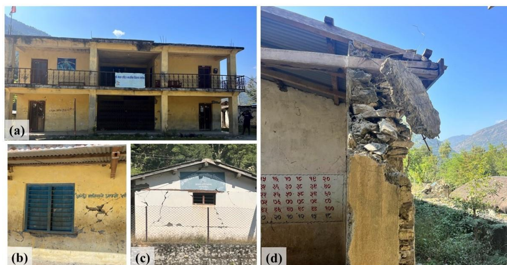
Figure 16. (a–d) Damage to school buildings of Jajarkot ( 28^{\circ}41'53'' N, 82^{\circ}16'20'' E) and West Rukum ( 28^{\circ}47'06'' N, 82^{\circ}18'55'' E).
