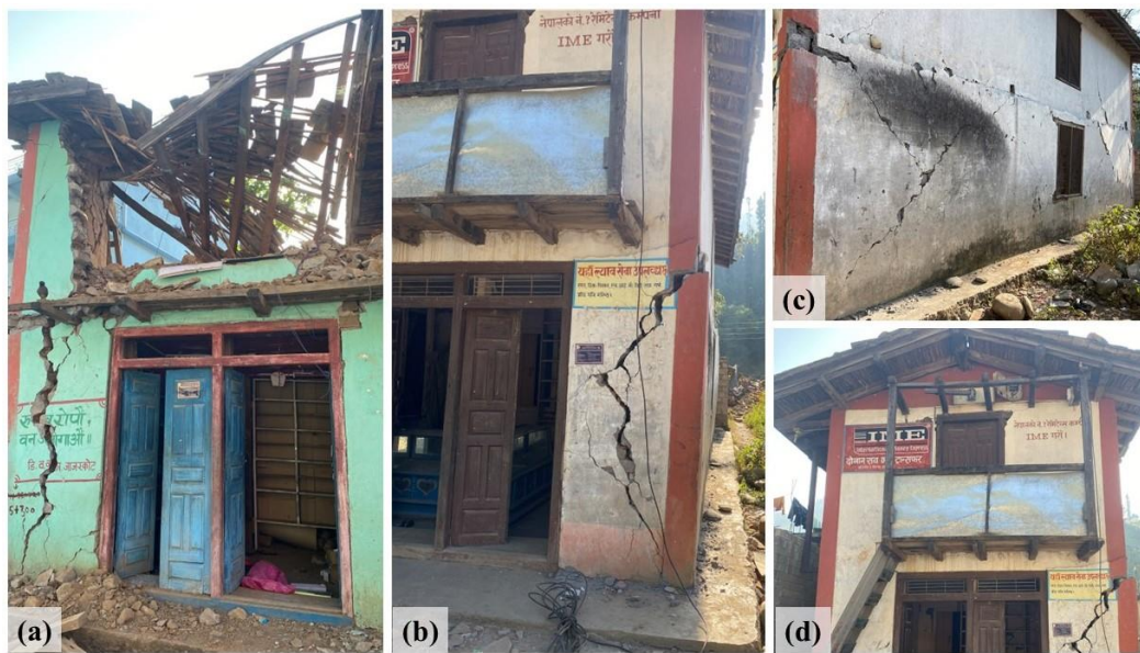
Figure 12. Damage in masonry buildings: (a) collapse of roof and failure of supporting walls of the building; (b) failure at the corner; (c) diagonal cracks; (d) vertical separation of masonry pier at corner ( 28^{\circ}41'57'' N, 82^{\circ}16'44'' E).
