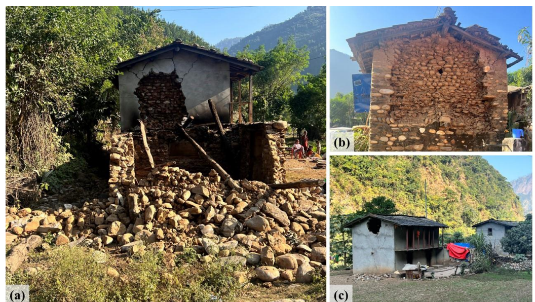
Figure 13. Damage in masonry buildings: out of plane collapse of stone masonry wall (a) ( 28^{\circ}41'56'' N, 82^{\circ}16'46'' E) (b) ( 28^{\circ}41'54'' N, 82^{\circ}13'45'' E) (c) ( 28^{\circ}42'42'' N, 82^{\circ}16'59'' E).
