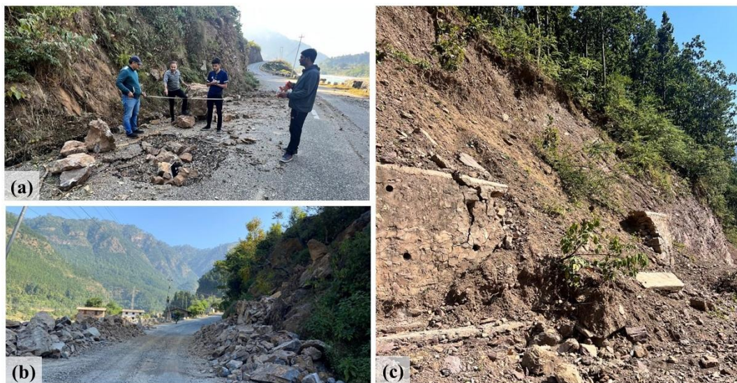
Figure 22. Damage in road infrastructure: (a) rockfall caused large size pothole in pavement, with maximum size up to 1.8 \times 2.3 \text{ m} ( 28^\circ 42' 17'' \text{ N} , 82^\circ 14' 08'' \text{ E} ) (b) road blockage due to rock fall ( 28^\circ 42' 29'' \text{ N} , 82^\circ 14' 17'' \text{ E} ) along Midhill Highway (c) failure of roadside slope retaining wall ( 28^\circ 48' 05'' \text{ N} , 82^\circ 17' 25'' \text{ E} ) along local road nearby Nalgad Bazaar.
