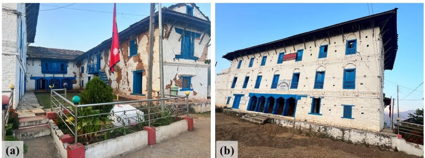
Figure 15. Damage to historical Jajarkot Palace, Khalanga, Jajarkot ( 28^{\circ}41'56'' N, 82^{\circ}12'01'' E) (a) plaster spalling with several diagonal cracks and (b) cracks on the wall.
