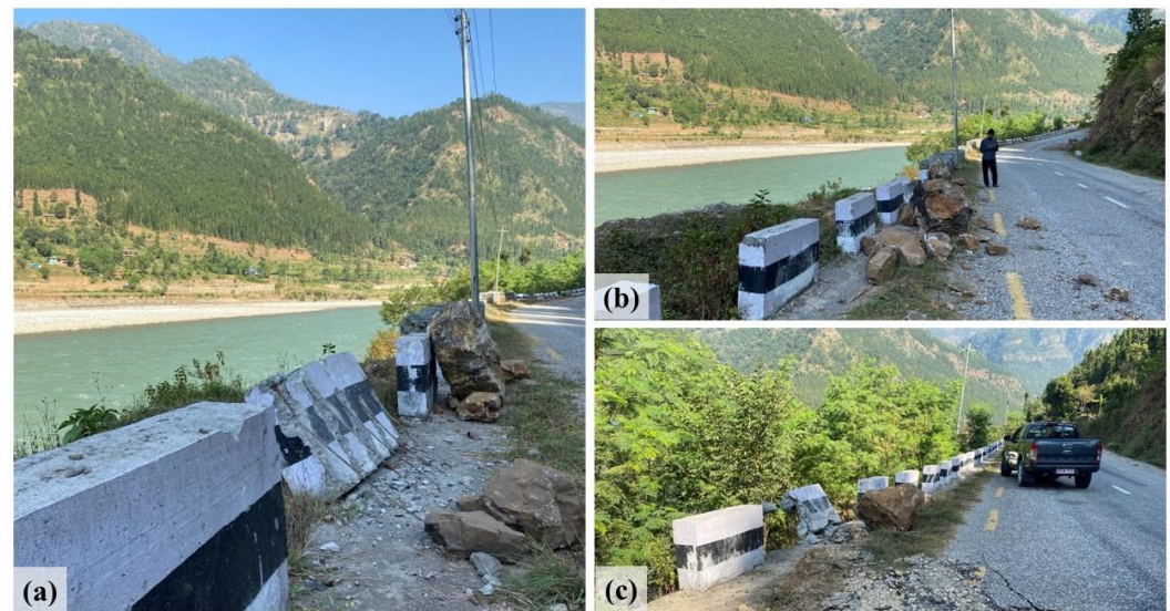
Figure 24. Damage to roadside concrete barriers in different sections along Midhill highway, West Rukum district (a,b) ( 28^{\circ}42'15'' N, 82^{\circ}14'07'' E) (c) ( 28^{\circ}42'17'' N, 82^{\circ}14'08'' E).
