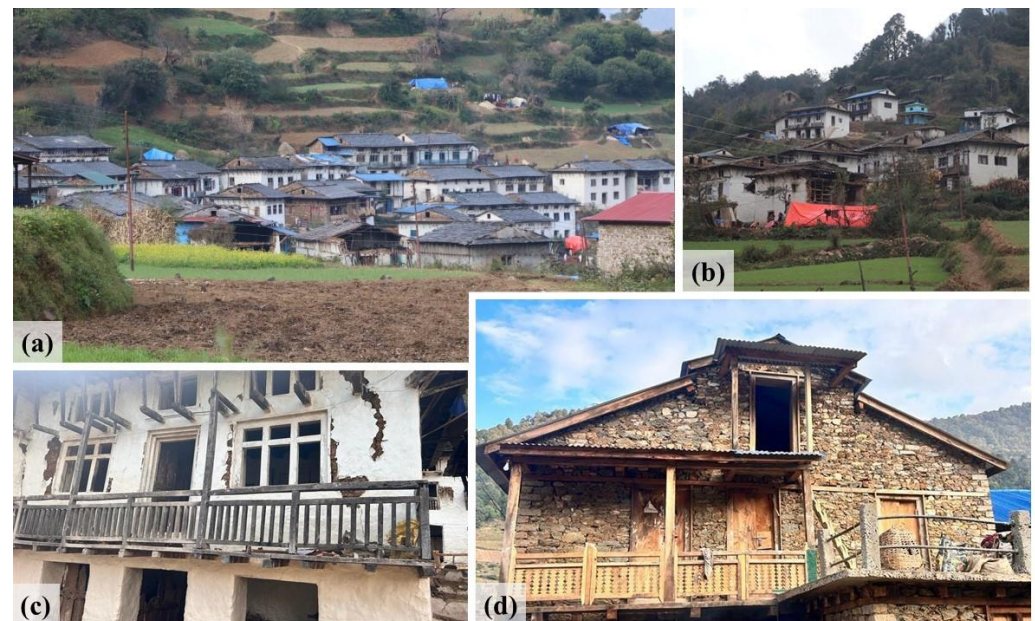
Figure 10. (a,b) Sherpa Village near the epicenter (Ramidanda); (c) vertical and joint shear cracks; (d) undamaged building with wooden bands (28°55′11″ N, 82°15′03″ E).
