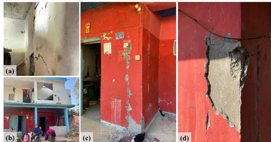
Figure 6. Damage to RC frame building: (a) cracks in the walls; (b) front view of the two-story building; (c,d) separation of column from the masonry infills ( 28^{\circ}41'55'' N, 82^{\circ}13'45'' E).
