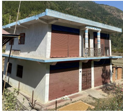
Figure 8. RC-framed building in West Rukum with no adherence to building code guidelines.
