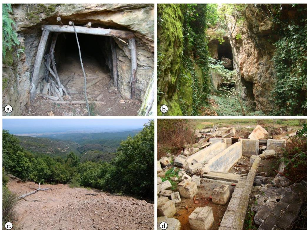
**Figure 4.** Photographs from the sampling survey: (a) The entrance of an old gallery; (b) A gallery parallel to the stibnite mineralization. Vertical wall rocks indicate the area of the exploited stibnite mineralization; (c) Waste material deposited downhill and opposite to a gallery entrance. (d) The destroyed flotation infrastructure near Zevgolatio village in the 1990s (Photo courtesy: Vasilios Melfos).
