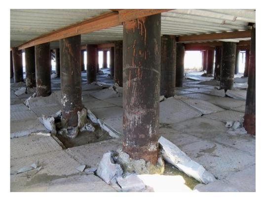
Figure 2. Piles affected by frost-heave uplift (gas field Zpolyarnoye, Western Siberia, Russia).
