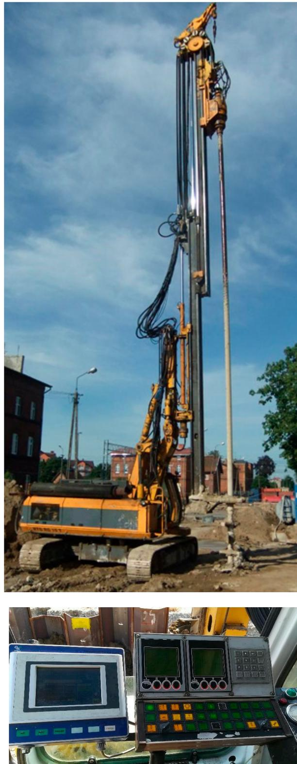
**Figure 2.** The machine used for performing Deep Soil Mixing (DSM) columns including the production parameter logging system.
