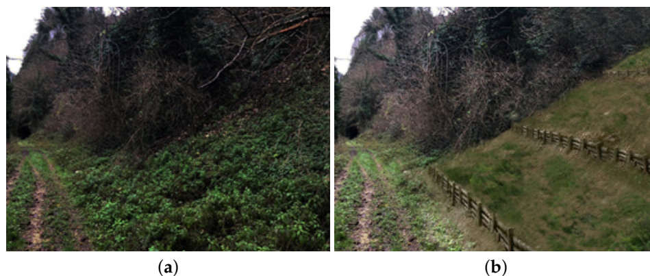
Figure 10. Simulated naturalistic work for S2 through photographic rendering: (a) initial condition of the slope; (b) condition after naturalistic work realization.
