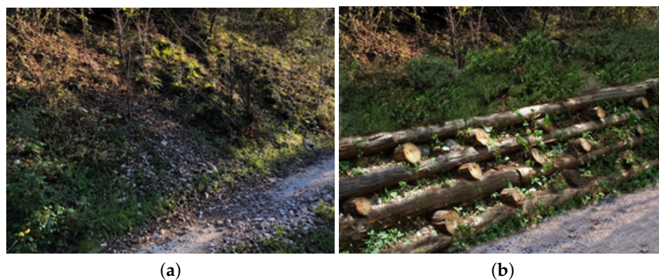
Figure 8. Simulated naturalistic work for S1 through photographic rendering: (a) initial condition of slope and (b) condition after naturalistic work realization.
