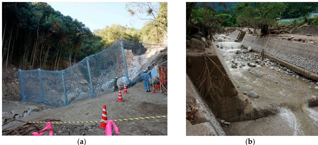
Figure 19. Examples of hard countermeasures of sediment disasters. (a) Steel net for capturing small debris flow, (b) Channel work.
