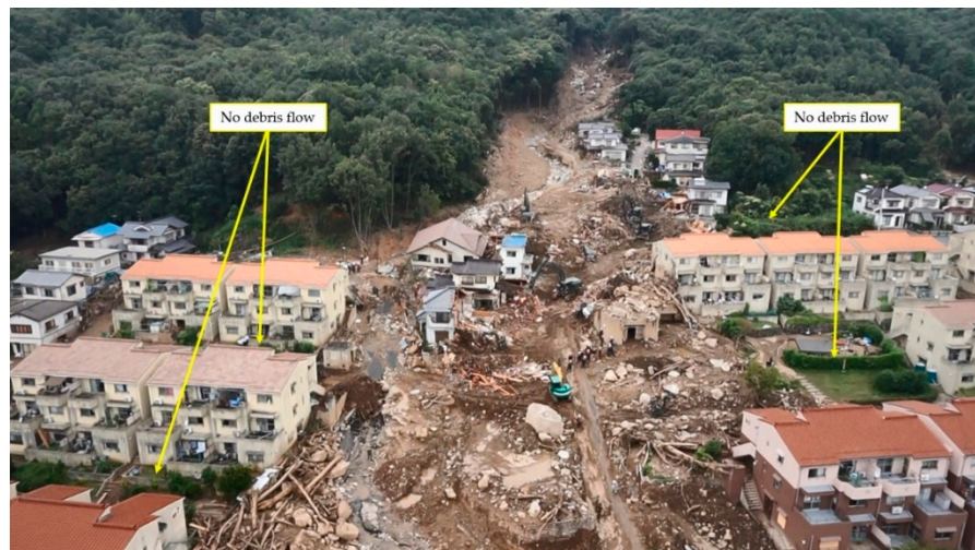
Figure 12. Debris flow no-inundation areas in the downstream reinforced concrete building area. Photo was taken by Luce Search Inc.
