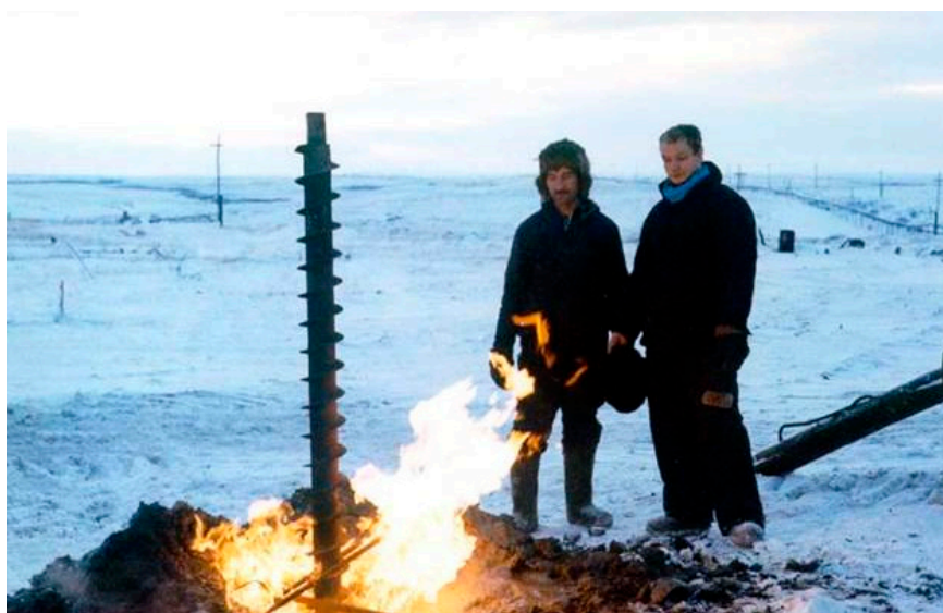
Figure 8. Methane emission from depths of 20–30 m during drilling of geotechnical boreholes in Pelyatka gas–condensate field (Gydan Peninsula, number on the map: 17).
