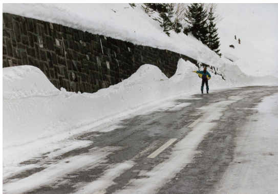
Figure A4. Traces of the deposit of the non-dense part of the Scex Rouge avalanche on the pass road after it was cleared. The railing was probably hit by a rock transported by the avalanche. Rocks up to 1 ton reached the road in the 1981 event.
