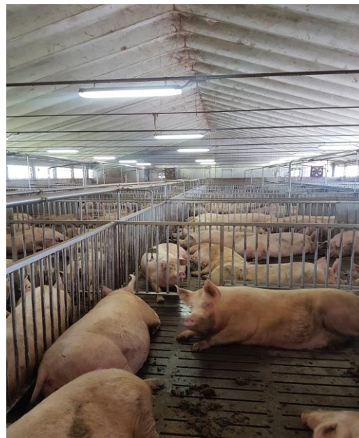
Figure 4. A mixed ventilation system in a piggery, characterized by natural ventilation in winter and mechanical fans in summer.
