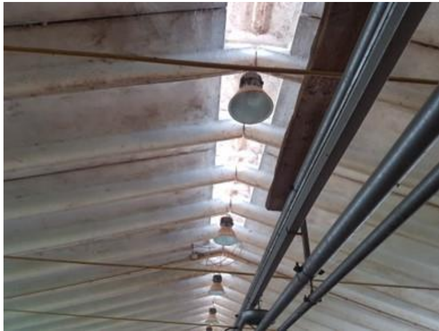
Figure 2. In a natural ventilation system, the opening in the roof ensures air exchange in a piggy.
