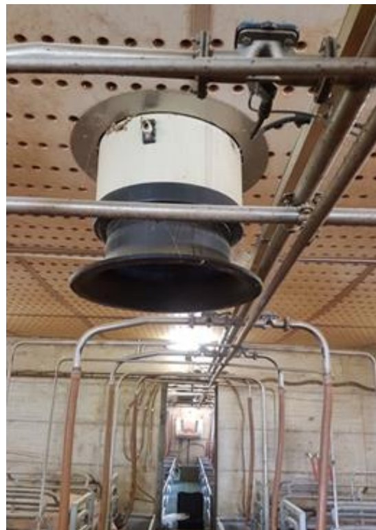
Figure 3. A mechanical fan guarantees the air exchange in an accurate way, according to thermal animal requirements.
