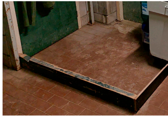
Figure 5. Example of a basic hygiene lock design at the entrance of a poultry building (taken from inside the anteroom towards the entrance door of the poultry building), as applied by many poultry farms in the Netherlands: separation of the dirty and clean area using a wooden board construction; at this point, one would change personal footwear for farm footwear; on the left side, the door towards the shower and toilet.
