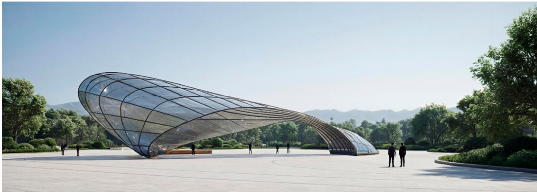
Figure 5. Visualization of the freeform pavilion—curved panelization. Source: author.
