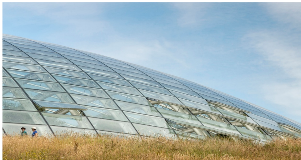
Figure 10. The Great Glasshouse, a curvilinear glasshouse structure with flat quadrangular divisions, designed by Foster + Partners, 2000.
