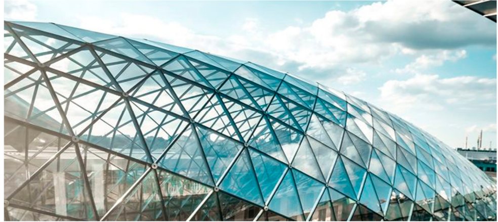
Figure 9. DG Bank, curvilinear surface with mesh triangular panelization, designed by Frank Gehry, 2001.
