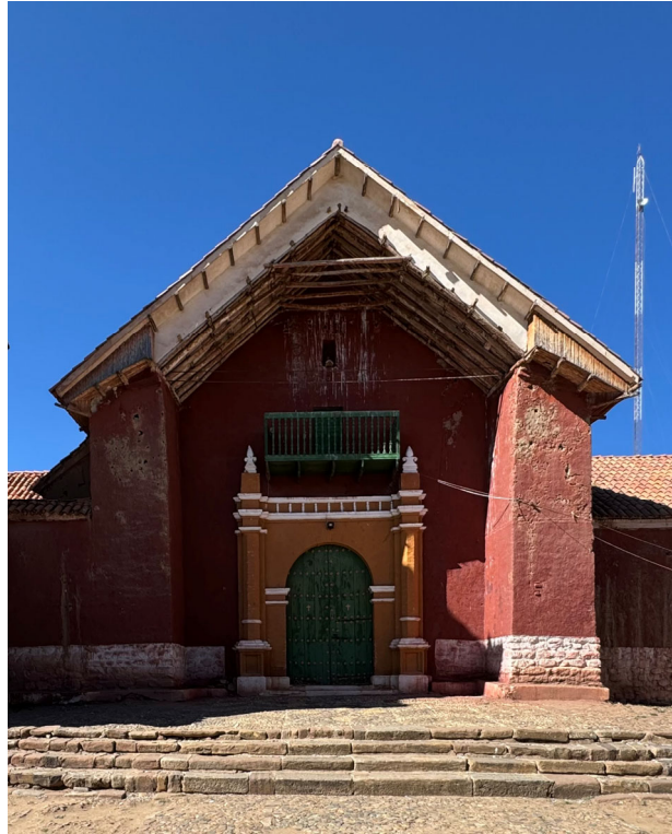
Figure 18. Façade of the Church of San Bartolomé, Carabuco, Bolivia. Photo by the author.
