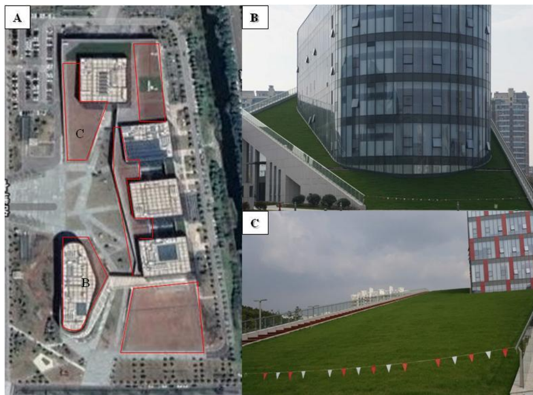
Figure 1. Photos of the green roof project. (A): Map of TongZhou Civil Squares; the red lines indicate the green roofs constructed using centipedegrass; (B): Slope green roof (27%) on the building of the Culture Center; (C): Flat green roofs on the buildings of Women and Children Center, Archive, and Library and a slope green roof on the building of Citizen Service Center.
