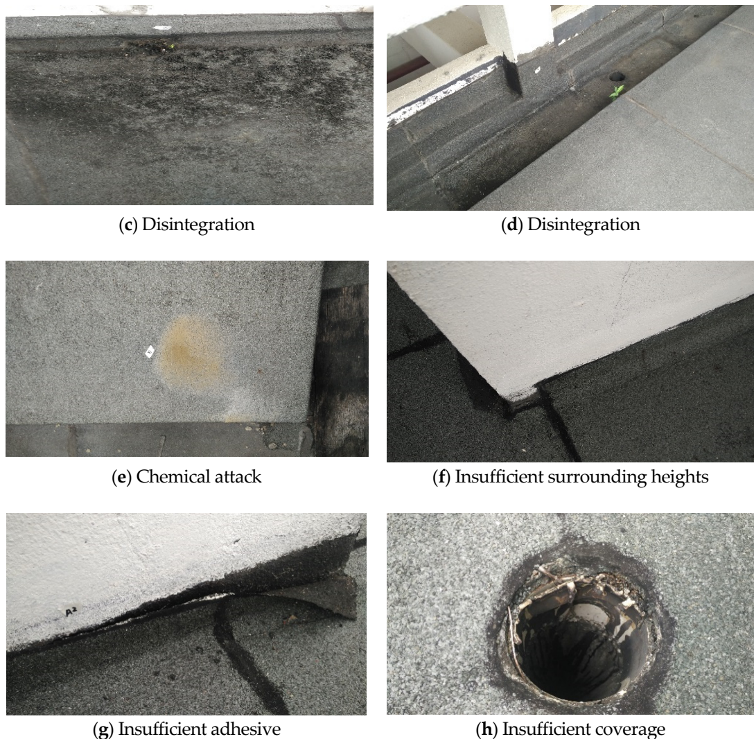
Figure 10. Defects identified in remedial treatment.
