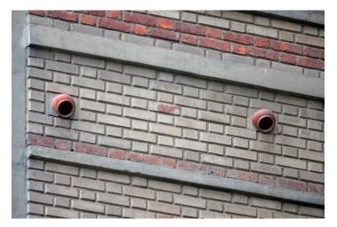
**Figure 27.** Clay pots inserted randomly into the external walls of DA building offer nesting places for birds and bees (Photo: Author).
