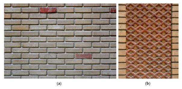
**Figure 28.** The material palette of the DA building consists of earthy materials such as (**a**) cement-stabilised compressed-earth blocks and (**b**) terracotta tiles (Photos: Author).
