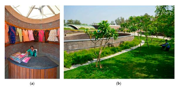
**Figure 34.** (**a**) Tensile canopies with ceiling fans cover the craft shops; (**b**) large usable green roofs above air-conditioned shops (Photos: Author).
