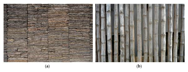
**Figure 35.** Cladding materials used in Dilli Haat Janakpuri: (**a**) Delhi Quartzite Stone and (**b**) bamboo (Photo: Author).
