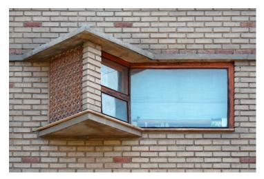
**Figure 26.** Window on the west façade having a prism-shaped protrusion to block the afternoon summer sun (Photo: Author).
