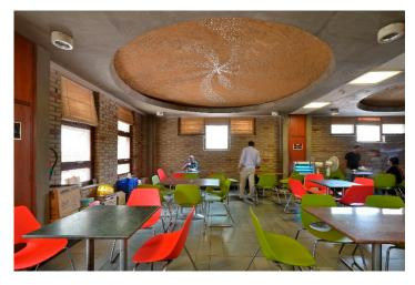
Figure 24. Shallow domed ceilings span the interior spaces of the DA building (Photo: Author).
