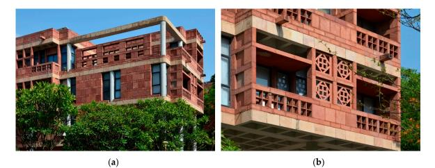
**Figure 10.** (a) Sandstone clad external skin delays heat transfer into the CIET building; (b) balconies and *jaali* screens protect the rooms of the CIET building from direct sun (Photos: Author).
