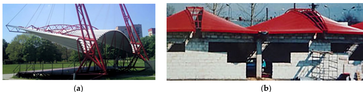
Figure 3. Two transformed free-form roof structures composed of a few warped shells: (a) an amphitheater on the boulevards and (b) a number of stores.
