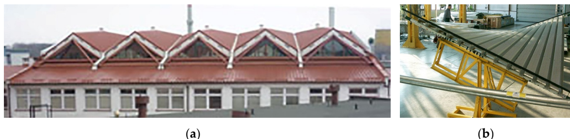
Figure 1. Transformed sheetings: (a) an erected complex roof structure of many hyperbolic paraboloid shells and (b) an experimental folded shell.
