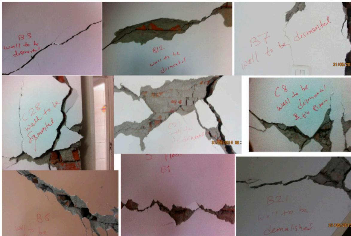
Figure 6. Infill wall damage due to Gorkha earthquake in the case study building.
