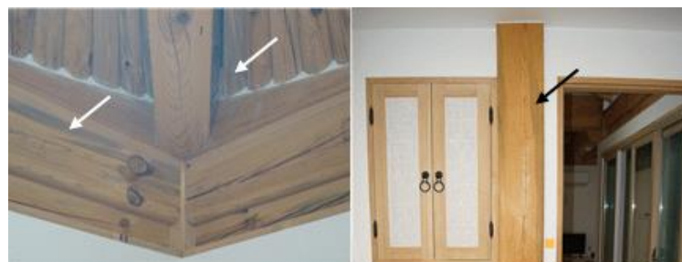
Figure 6. Hanok defects: bluish changes.
