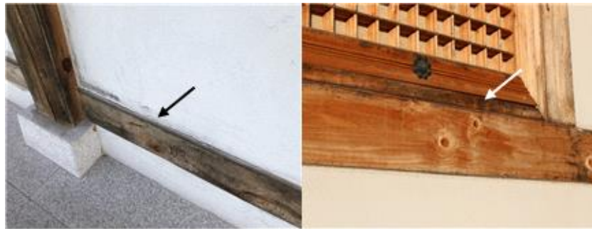
Figure 5. Hanok defects: fungal generation and discoloration.
