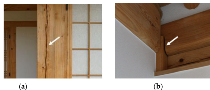
Figure 8. Hanok defects: parallel twists and joint fissures. (a) Parallel twists; (b) Joint fissures
