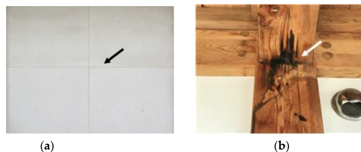
Figure 9. Hanok defects: parallel twists and joint fissures. (a) Wall cracks; (b) Adhesive elution
