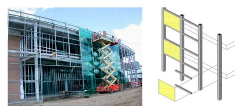
Figure 3. Stick Built Curtain Wall [12].
